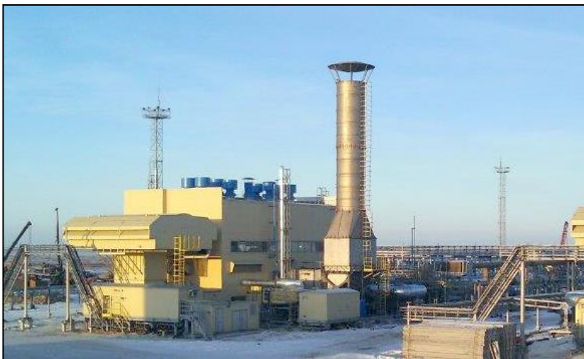
Compressor Booster Station at the Yurkharovskoye field
